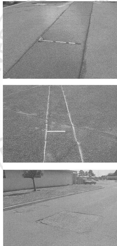
Gambar 2. 22 Tambalan ( Patching and Utility Cut Patching )
