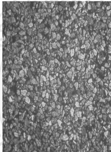
Gambar 2. 24 Pengausan Agregat ( Polished Aggregate ) Sumber: M.Y. Shahin 1990
