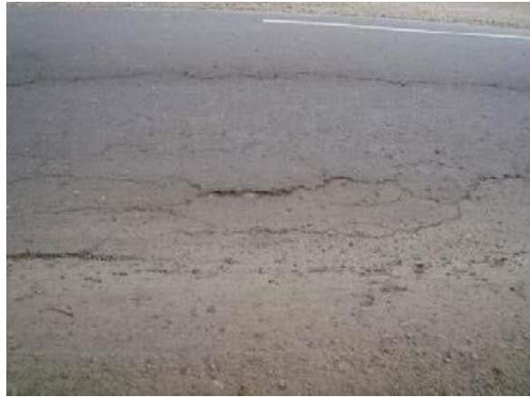
Gambar 2.5 Cekungan (Bumps and Sags)
