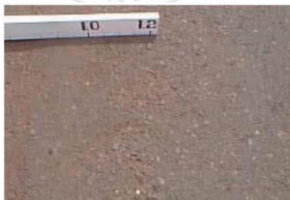
Gambar 2.13 Pengausan Agregat ( Polished Aggregate )
