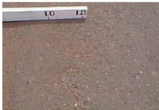
Gambar 2.13 Pengausan Agregat ( Polished Aggregate )
