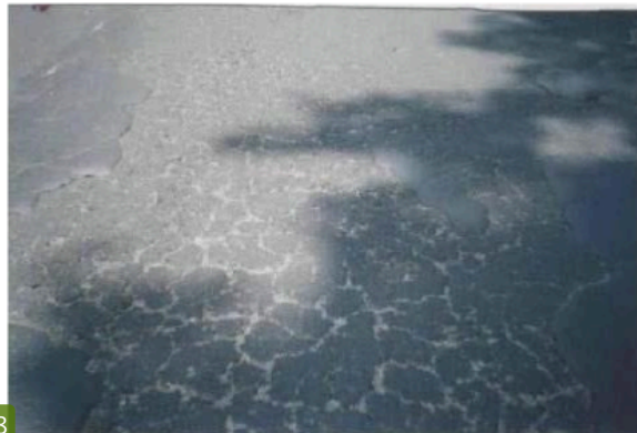
Gambar 2.20 Pelepasan Butir (Weathering/Ravelling)
