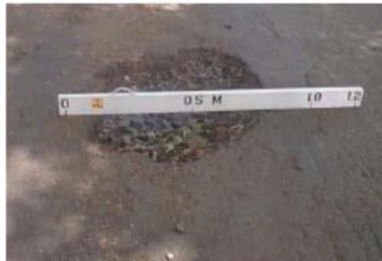
Gambar 2.14 Lubang ( Potholes )
