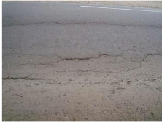
Gambar 2.5 Cekungan ( Bumps and Sags )
