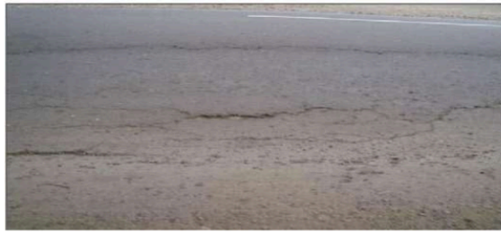
Gambar 2. 7 Cekungan (Bump and Sags)
